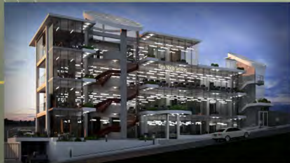
New Media Services Office Building PEZA, Baguio City
